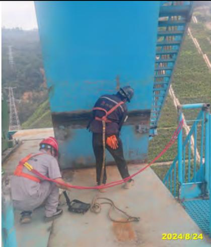
A photograph showing two workers in safety gear (hard hats, safety harnesses) performing ultrasonic testing on a blue steel structure. One worker is kneeling and using a device, while the other stands nearby. A red safety rope is visible. The date '2024/8/24' is printed in the bottom right corner of the image. |
