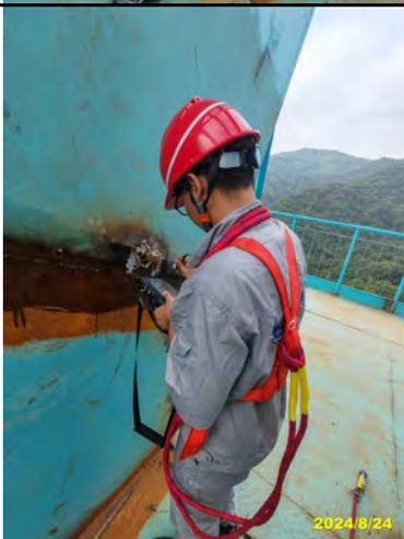
A worker wearing a red helmet, safety glasses, and a grey safety harness is performing ultrasonic testing on a blue-painted steel structure. The worker is holding a device and looking at the results. The background shows a hazy landscape with hills. A yellow timestamp '2024/8/24' is visible in the bottom right corner of the photo. |
