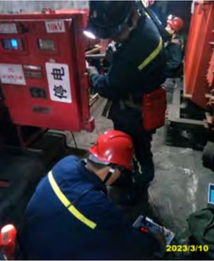
A photograph showing workers in blue uniforms and red hard hats inspecting a large red high-voltage switch cabinet. The cabinet has a '10kV' label and a '停电' (Stop Power) sign. The workers are using tools and equipment to perform the inspection. A date stamp '2023/3/10' is visible in the bottom right corner of the image. |
